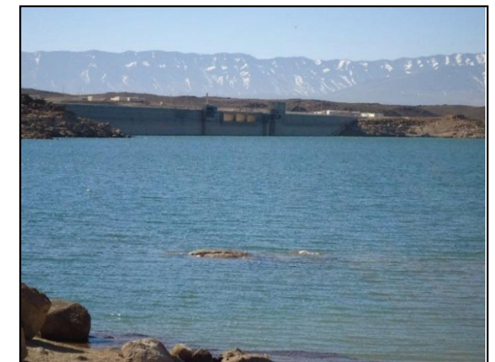
Photo 8 Hassan II dam
